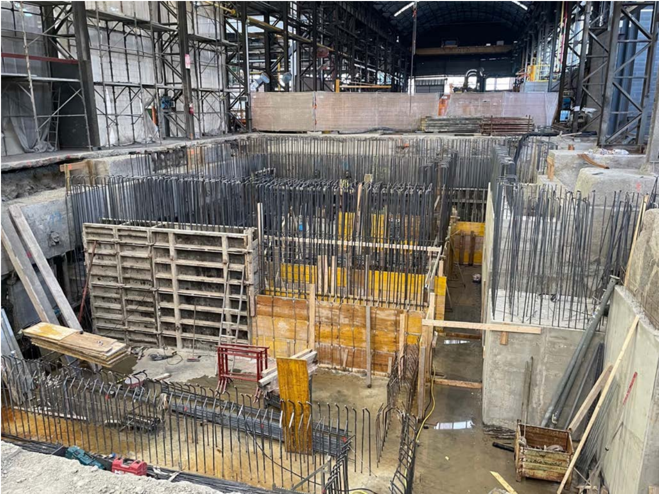
Oggiono Plant - Foundations for the installation of the new rolling mill
