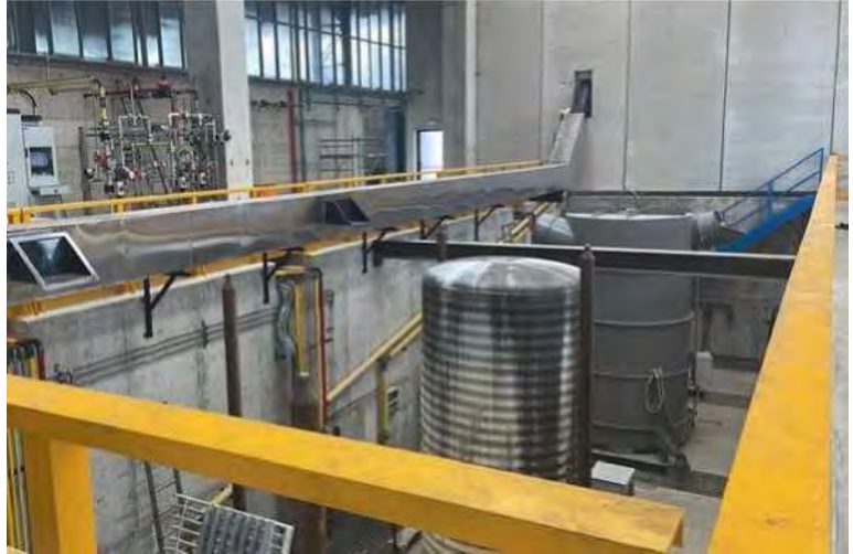
Oggiono plant - New pit for furnace revamping
