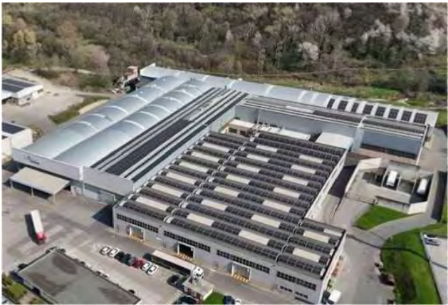
Oggiono building - 1MWH photovoltaic system
