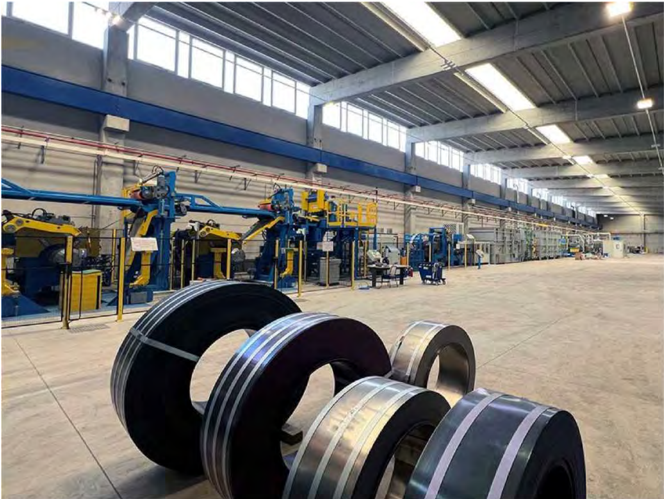
Oggiono plant - Hardening and tempering line
